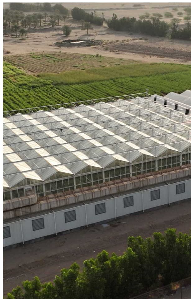
Glass and air-conditioned greenhouses using the latest technologies to control the internal environment of the farm, Mishkat
